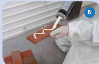
6 Apply adhesive to rear of slip
