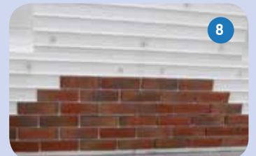
8 Build up wall to required bond pattern
