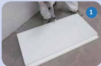
1 Apply adhesive to panel and adhere to substrate
