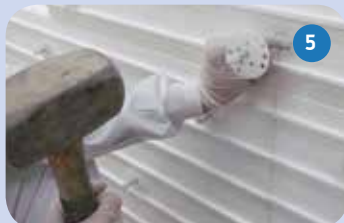
5 Secure panels with fixings
