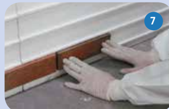
7 Press brick slip into position
