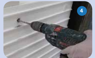
4 Prepare substrate for fixings
