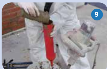
9 Fix mortar in bucket, fill hand pump
