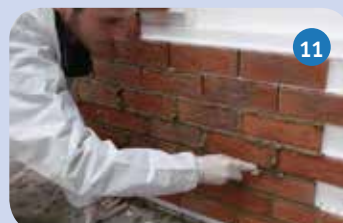
11 Strike joints before tooling
