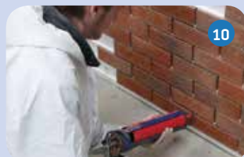
10 Apply to joints and over fill
